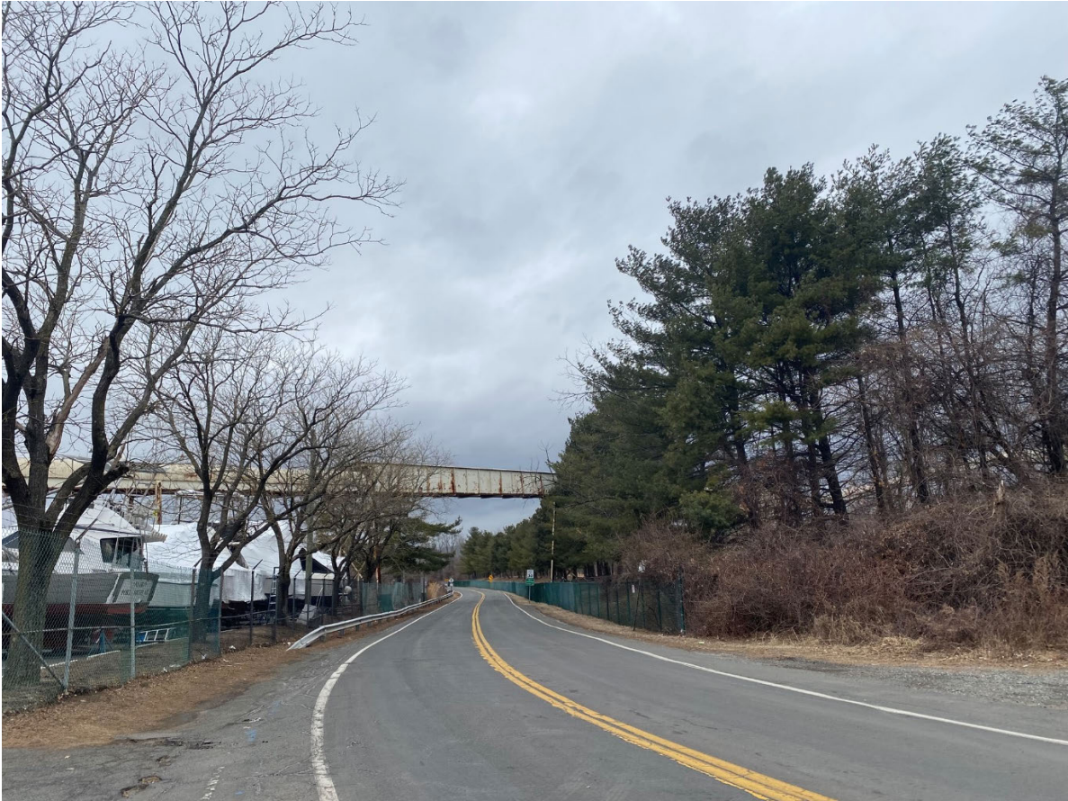
Conveyor over Beach Road (Marina boat storage on left of photo, gypsum plant behind evergreens on right)
