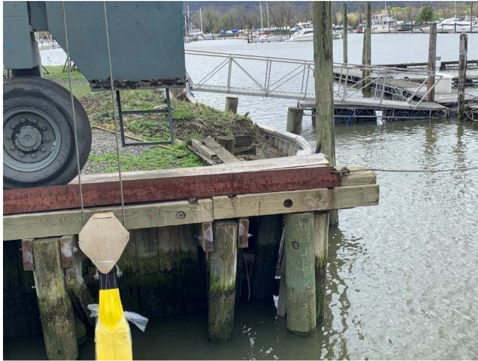
Bulkhead buckling
